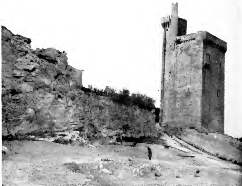
"THE TOWER OF PHILIP THE FAIR."—VILLENEUVE-LES-AVIGNON.
